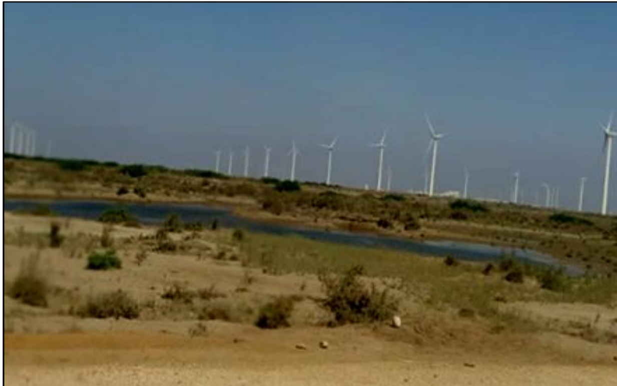
Fig. 5. Wind Turbines installation area.
